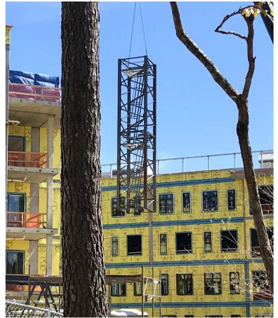
Removing last section of the mast
