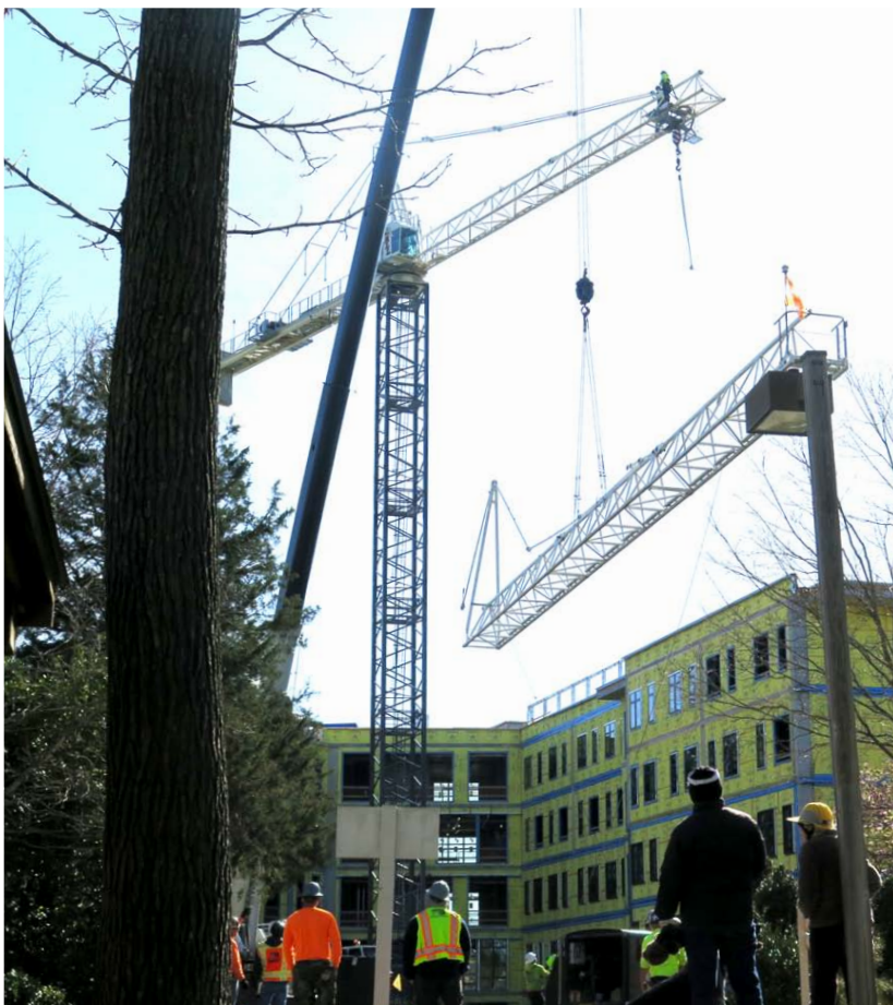
Removing a section of the large jib
