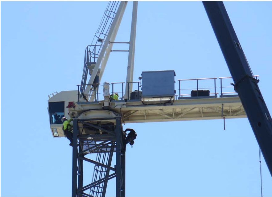
Slewing unit ready for removal from top of mast
