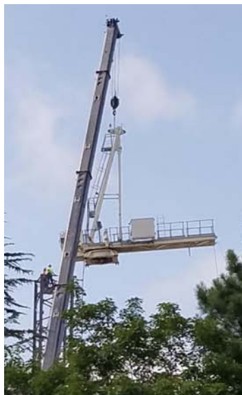
High-altitude assembly of the Tower Crane
