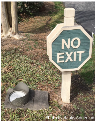
Abandoned upward-facing luminaire on TFAD Drive
