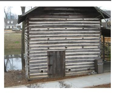
View of our south barn showing five tiers of dark beam ends—4 feet apart horizontally and 2 feet vertically (most in the bottom tier are missing). The top tier is just under the eaves, the lowest a yard above the floor. (A typical working barn would show matching beam ends on the opposite side of the building.) Sticks of tobacco were laid across these beams to be cured by a floor-mounted heating system. The large holes near the bottom are vents.
